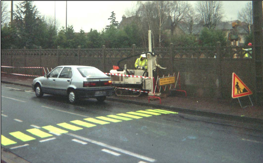
Photo 1 : Geoprobe on Drilling location
